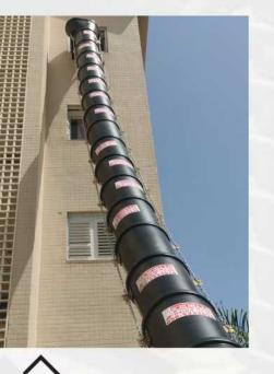
The debris chute is used in construction to neatly funnel trash from different floors of a building through a column in order to avoid accidental damage to workers or pedestrians.
